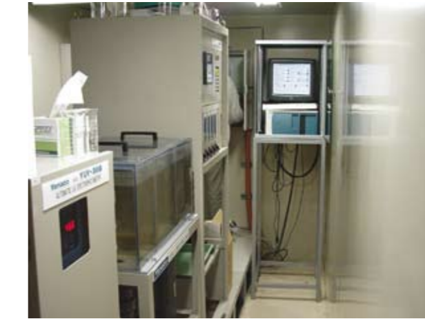
Inside the monitoring station
